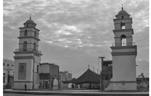
Church in main square of Pisco. It collapsed during the earthquake, leaving only the bell towers.
